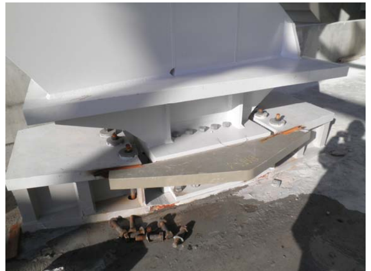
Lyon Stadium - General View –Spherical bearings between metallic pier and concrete support
