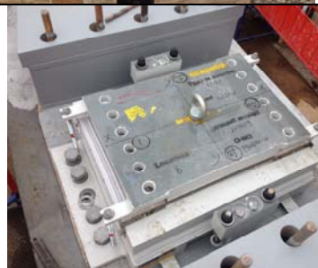
General design with uplift device and sliding plate below the Spherical part of the bearing
