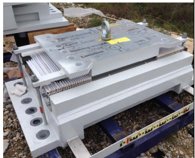
Lyon Stadium - General View –Spherical bearings between metallic pier and concrete support
