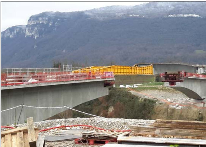
Central Metallic Span between the two concrete cantilevers
