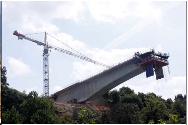
Lateral Concrete Cantilever
